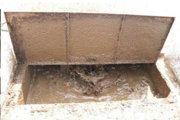
Mixing unit Size: - 5'9" X 5'9" X 2'6"
