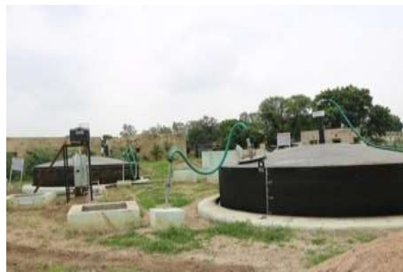
Two Digester: 60 m 3 Bio-gas Production per Day Each Digester
